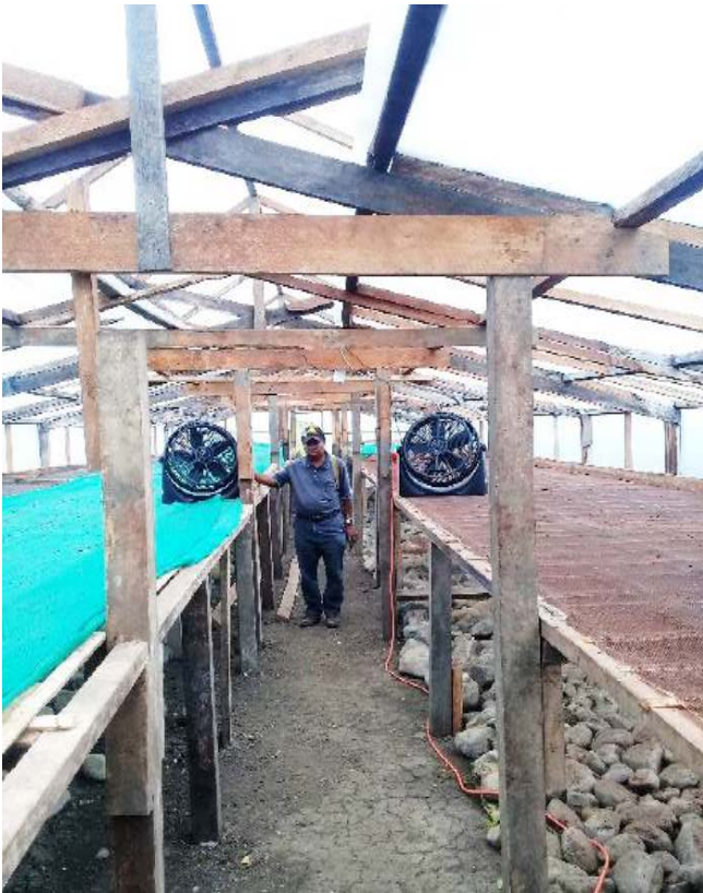
Figure 8: David Yinil alongside the solar-powered fans inside solar dryer at Yekimbole
