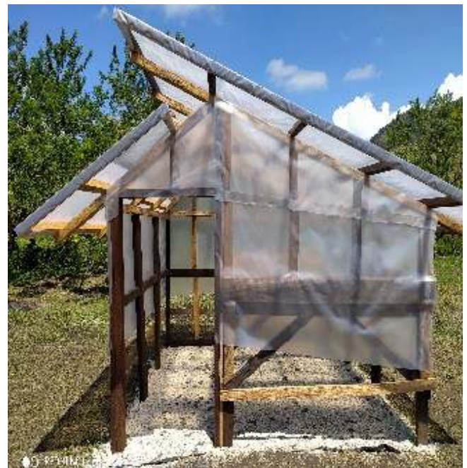
Figure 6: Simple design solar drier constructed in Sualu Village, Bogia District – another modification of the basic design.
