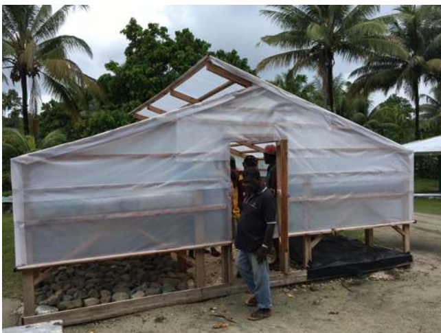
Figure 10: Cathy Miroi's just completed solar dryer, Luapul Village, New Ireland
