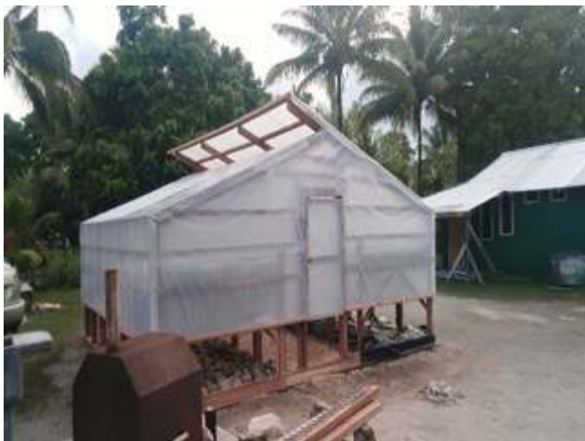
Figure 17 (below): Solar drier built at Luapul Village (CMFT Cathy Miroi), New Ireland.
