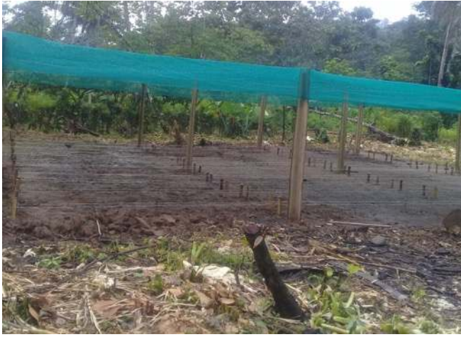
Figure 10 (above): Permanent nursery constructed at Torokina.
