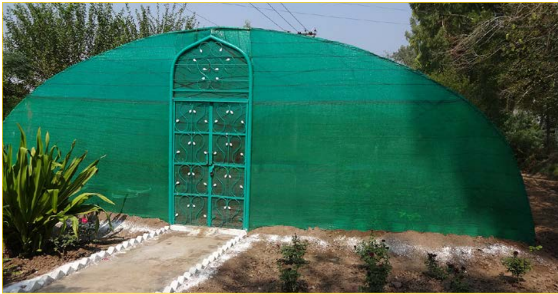
Figure 1.1 A modern citrus plant house in the Punjab.
